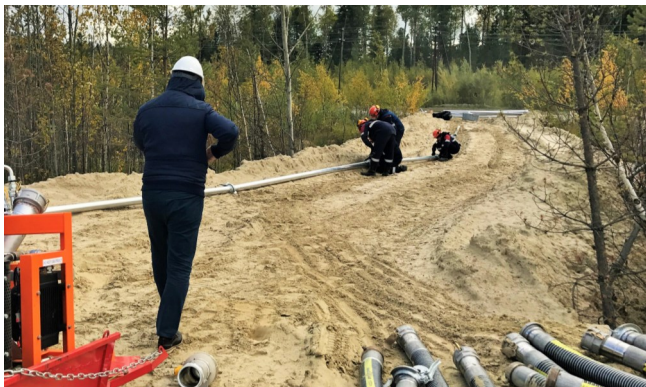
Mini Pipeline being assembled on site
