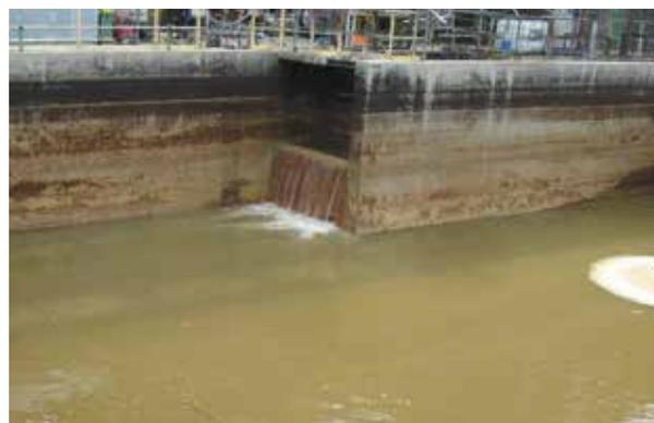
Tank cleaned of crust with Vikoma Crust Lance System
